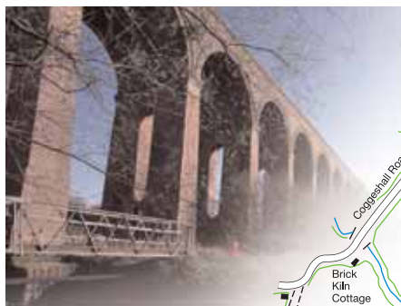
Chappel Viaduct, Chappel
